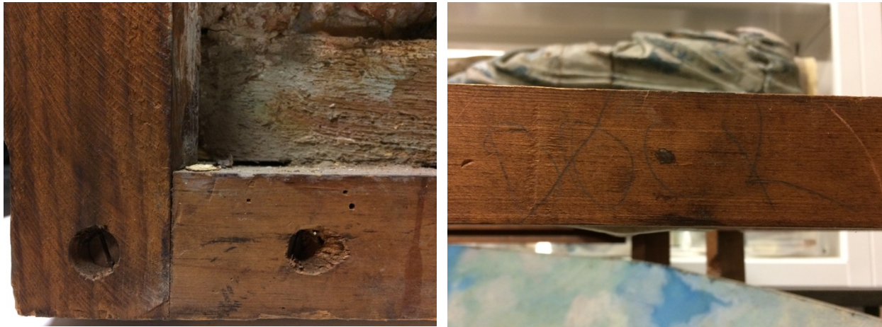
Fig 3 & 4. Detail of the mortised corner of the diorama's frame (not intended to be visible in exhibition) with screws and an un-sanded finish (left). Hand written "Dock" appearing on right of top beam of the recto of the diorama (right).
